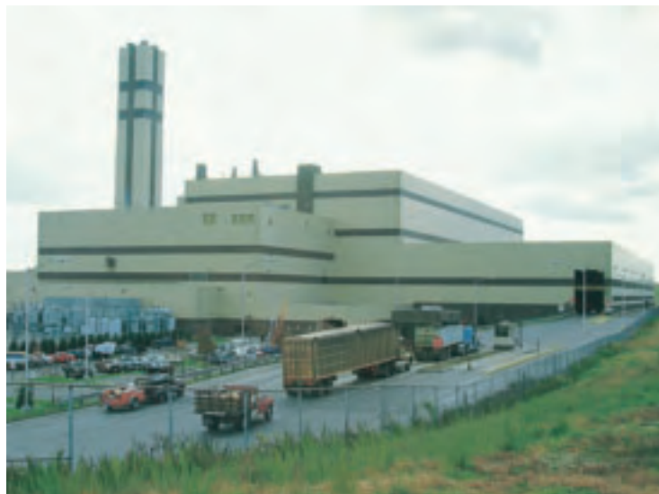
Figure 17 Garbage can be burned to produce electricity at trash-burning power plants such as this one in Virginia.
